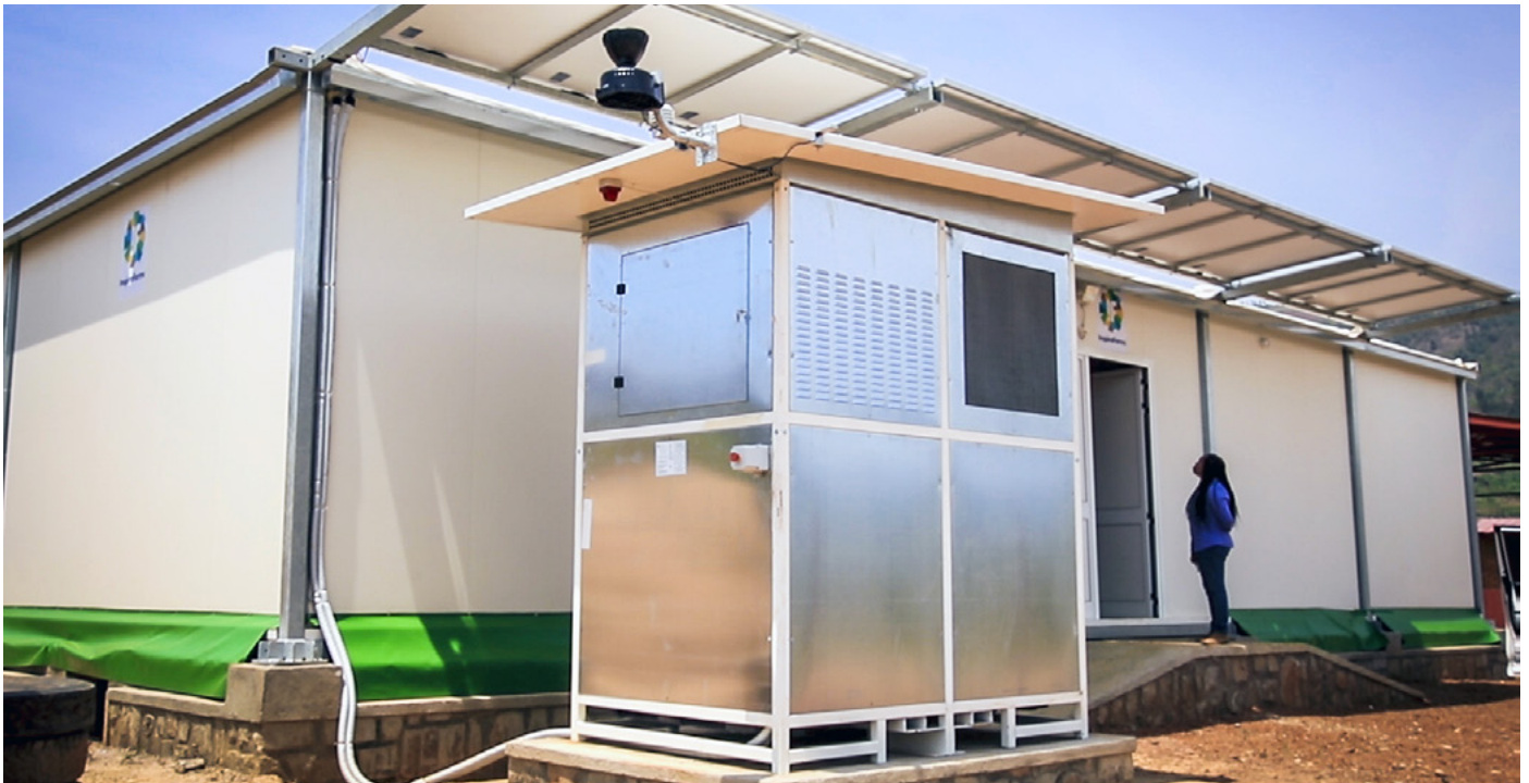
Figure 1: An off-grid cold-storage system designed by InspiraFarms, installed in Rwanda
