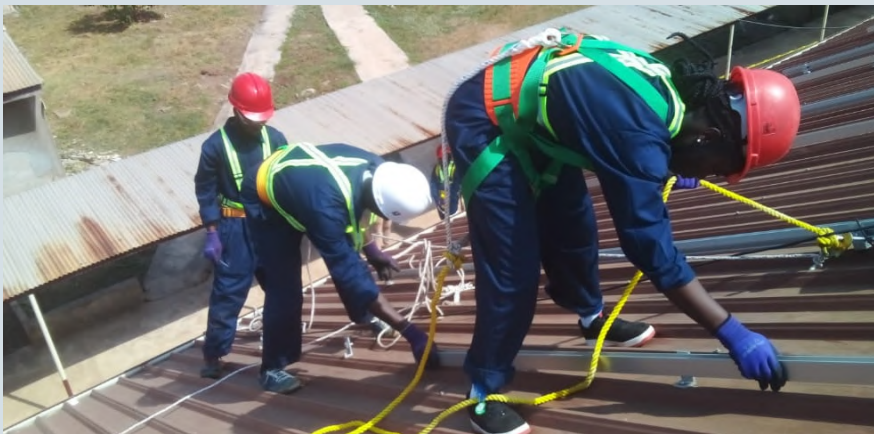
Figure 8 Installation of Stella Futura's system
