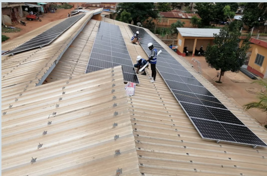
Figure 10 Installation of ARESS's system
