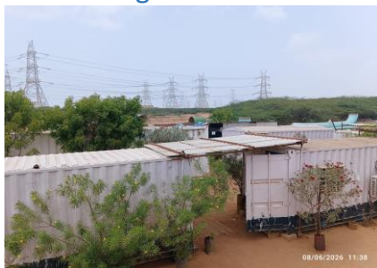
Cooling film applied on top of worker resting place. Source: SPACES field documentation
